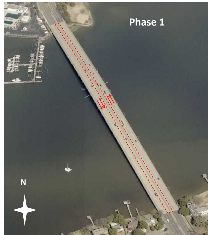
Phase 1 (Duration of approximately 3 months)
